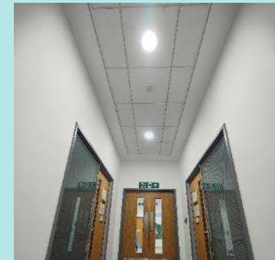
Newly installed LED downlights at Derriford
